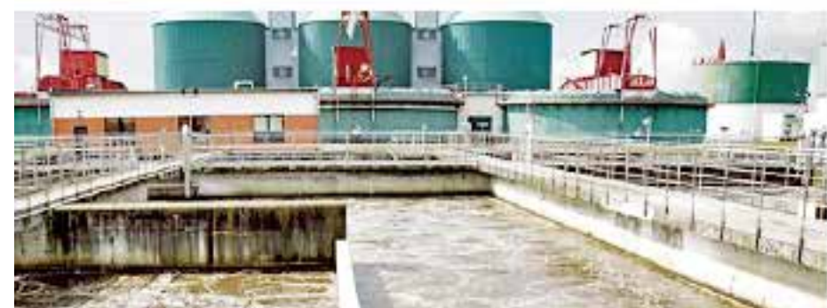
WASTE WATER TREATMENT
